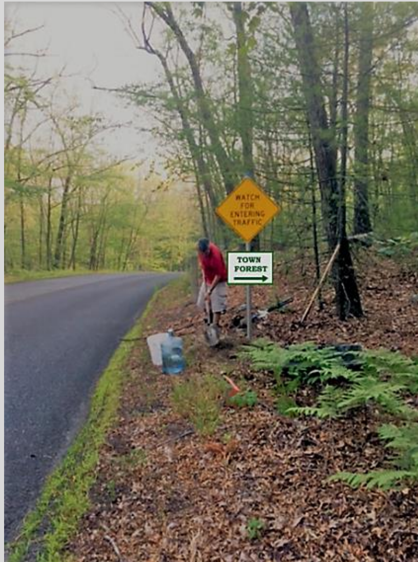
Town Forest Committee member and trail steward, Ryan Oliva, installs one of 2 signs alerting drivers of the entrance to the main parking lot just ahead along Millville Road.
