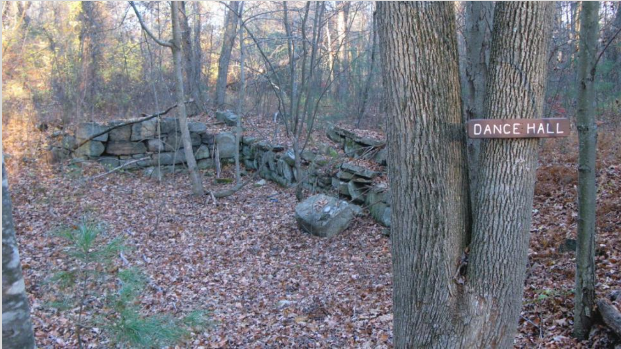
A portion of the foundation of the former dance hall and later grist mill as it appears today (2016). From the comparison of this photo with the one on the previous page, it appears much of the granite slabs have gone missing over the years.
